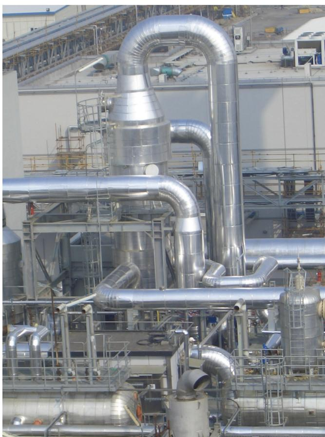
**Figure 2.** Vertical DDS unit in nitric acid plant.
